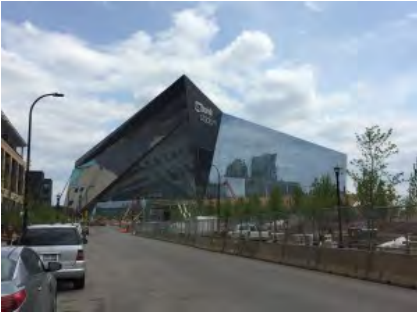
Stadium construction ahead of schedule
